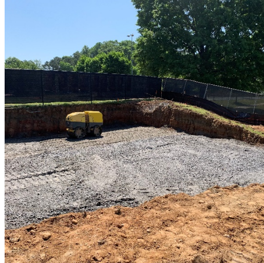
Backfill and Compaction
