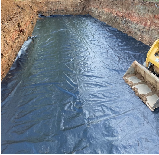
Geotextile Fabric in Place
