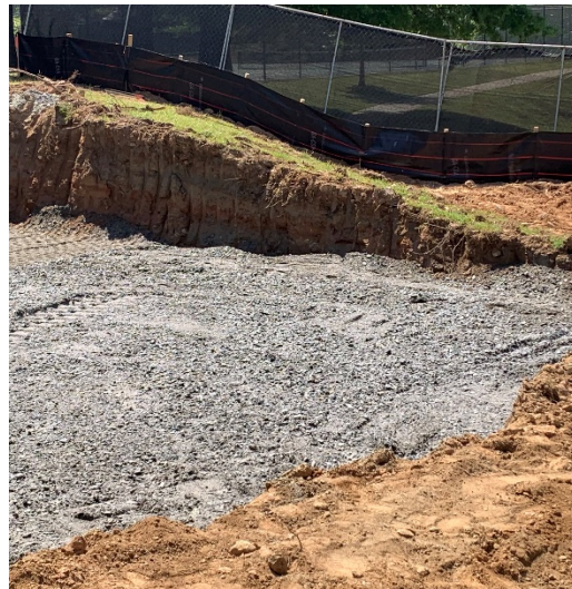
Backfill at East Elevation
